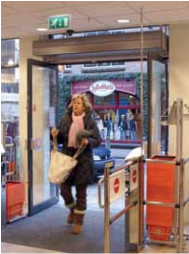
The DoorFlow above the door entrance creates a draught-free inner climate.
